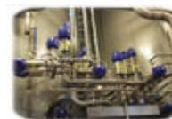
*Alfa Laval mix-proof valves with ThinkTop control are used in this dairy application. The controls indicate individual valve status, e.g., open and closed valve, seat-lift, solenoid status and maintenance. Source: Wayne Labs.*
